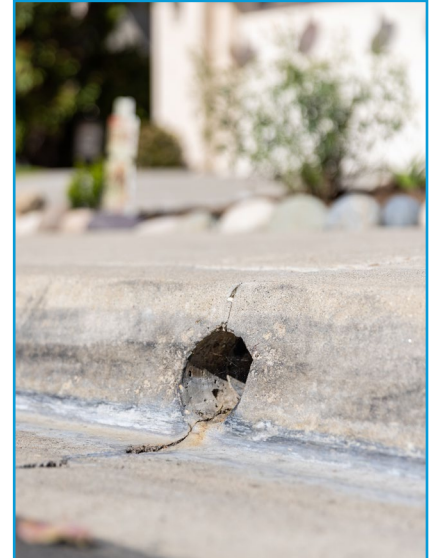
Curb cut with proper drainage.
